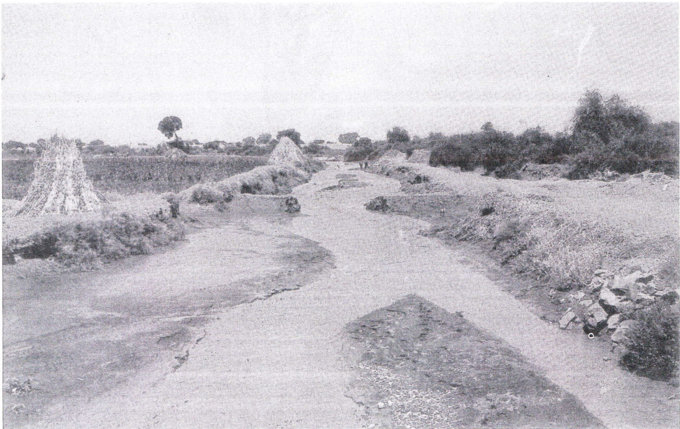
Silted canal - Headreach, Wadi Zabid system
